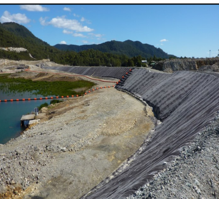
HDPE pipe and floats
