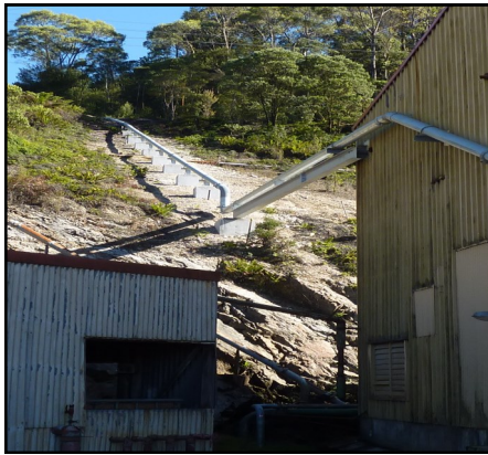
Steel pipe and pipe supports
